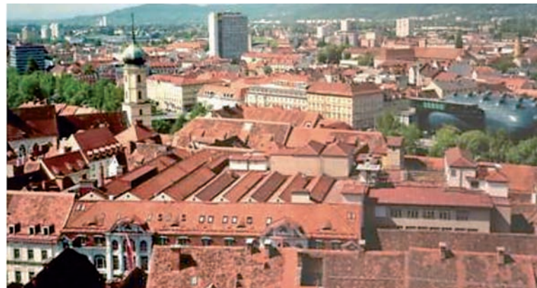
Graz, current state of the historic city centre
