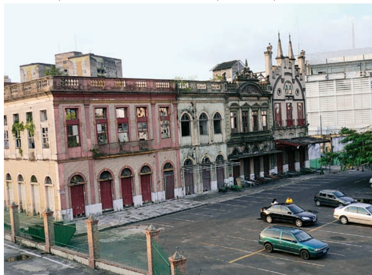
Manaus, dilapidated houses in the historic centre (Photo: M.Pz.)
