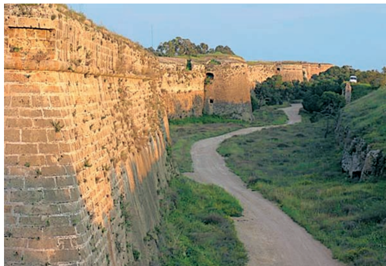
Fig. 6 The fortified walls and moat of Famagusta
