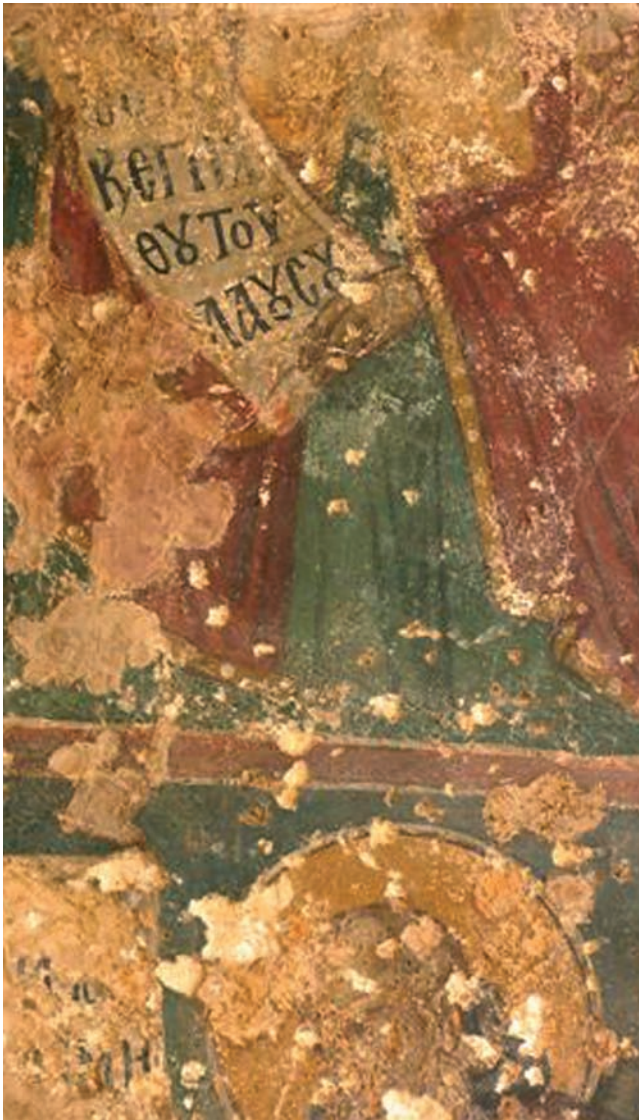
Fig. 17 Damaged frescoes in Saint George of the Greeks
