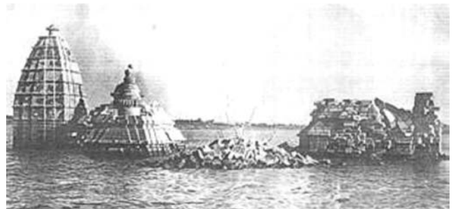
Temples 8, 9 and 10, partly submerged by Waters of river Damodar impounded by the Panchet dam. (West Bengal Directorate of Archaeology photograph, May, 1962)
