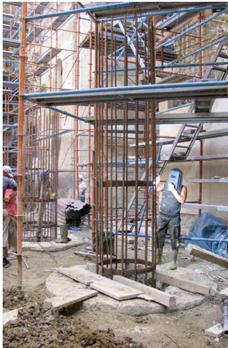
Authentic column bases perforated for the arrangement of concrete piles
