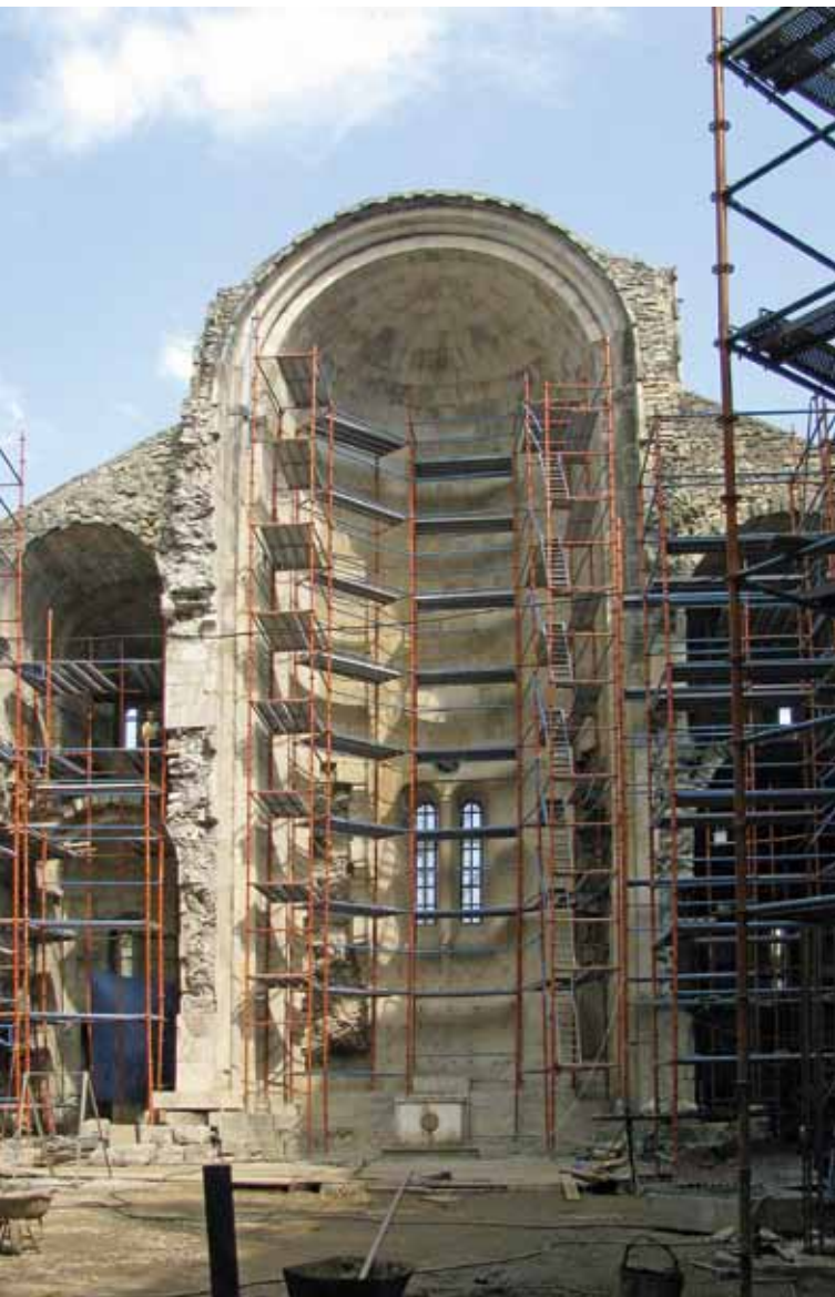
Bagrati Cathedral, the interior during reconstruction works in 2009
