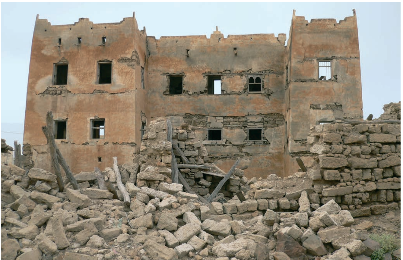
Mirbat, collapsed house of a rich merchant, Bayt al-Siduf (Photo: M.Pz.)
