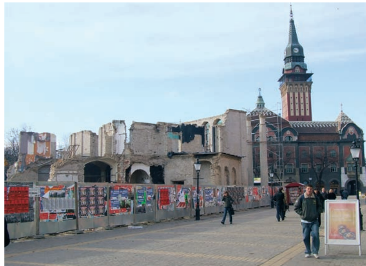
The theatre during the demolition in November 2007 ( www.kakanien.ac.at )
