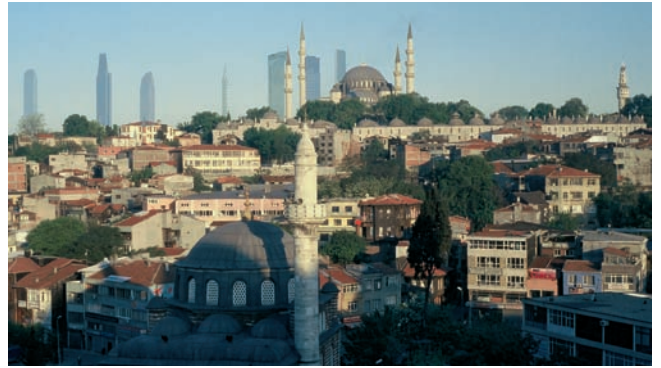
Fig. 11 Haydarpaşa and Süleymaniye Mosque seen from Zeyrek Terrace (simulation). The colossal Haydarpaşa site would appear from Zeyrek Terrace in the range of the Süleymaniye Mosque degrading the venerable silhouette and aura of the cupola and four slim minarets. (The Haydarpaşa towers are presented in a calculated scale). The Haydarpaşa Project will be visible from Galata Tower as well as from Galata Bridge and might even appear as a monster project in the view from Cihangir Mosque Garden. It was Yahya Kemal who in a poem perpetuated this famous view from Cihangir to Üsküdar at sunrise.
