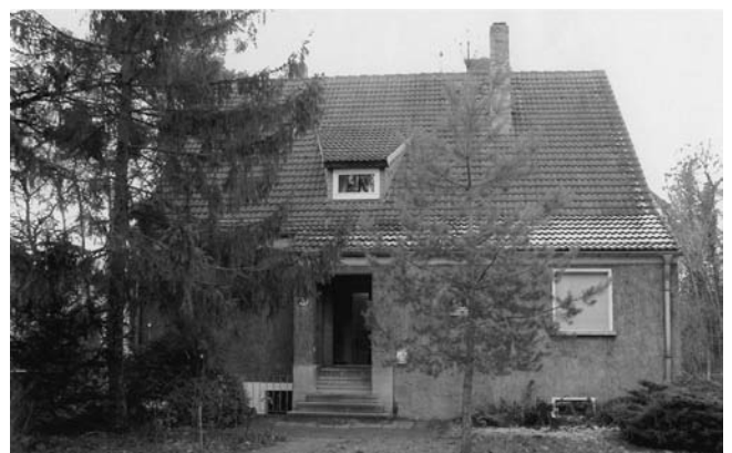
Dessau, former director's house, now "Haus Emmer", situation in 2004 (Photo: Stiftung Bauhaus Dessau)
