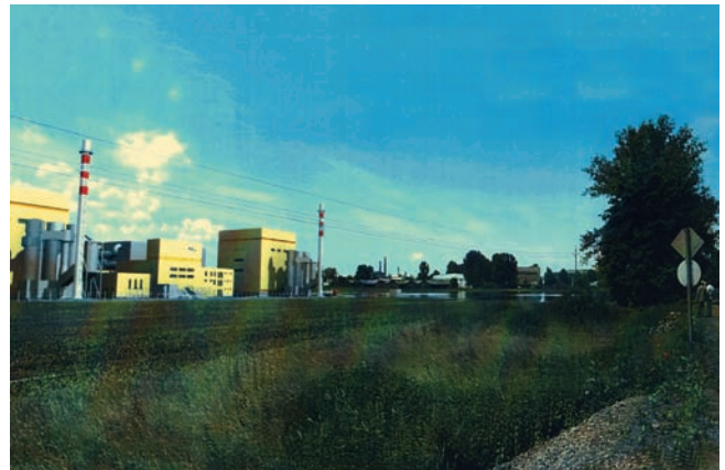
The first plan for the power station in the cultural landscape of Tokaj
