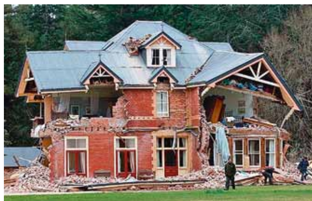
Christchurch, damaged private house
