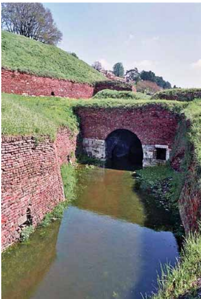
Belgrade Fortress, the walls during the flood
