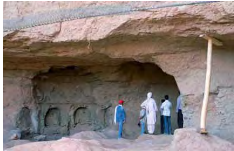
Parts of the niche's back wall had to be supported as stone slabs kept falling down
