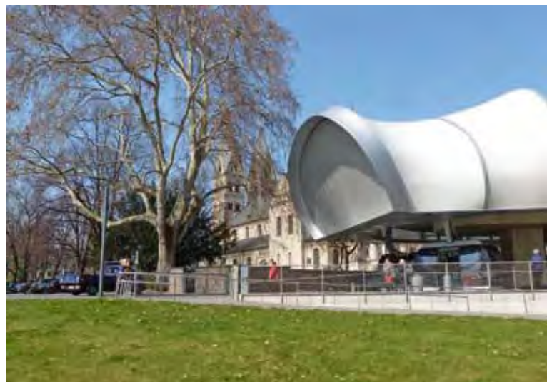
Cable car base station near the medieval church of St. Kastor (photo: C. Machat)
