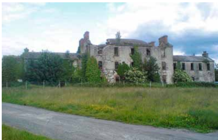
Former Military Barracks, Nenagh, Tipperary North, 2013
