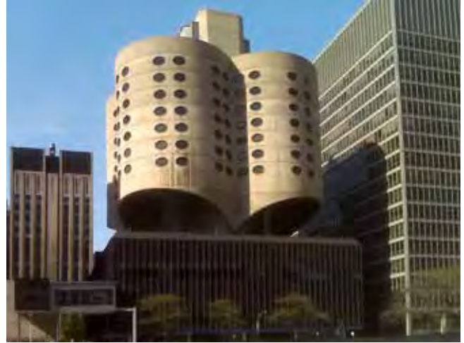
Prentice Women's Hospital, Chicago, Illinois (photo: courtesy of Landmarks Illinois)
