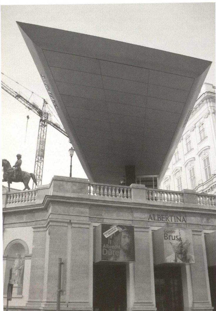
Vienna, Albertina, Museum of Graphic Arts. Fifty metre long overhanging roof, designed by the Austrian architect Hans Hollein, a symbol for the "roof-mania" in Vienna.
