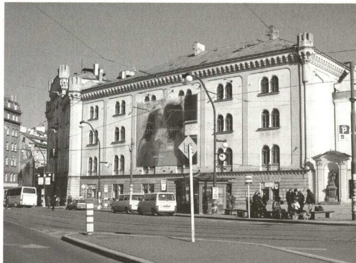
Prague, the historic Josefská Barracks from Republiky Square. The vacated building is ready for demolition. Only the façade is to be preserved.
