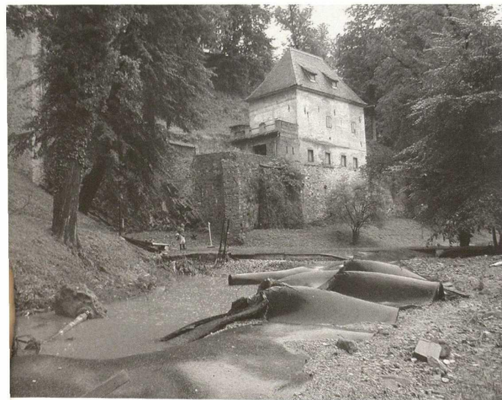
Ceský Krumlov, the brought down asphalt road in Jelenka
