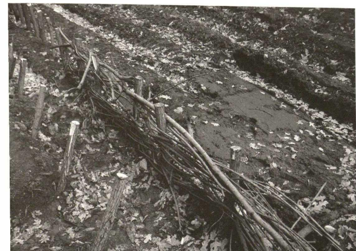
Kratochvíle, foundation of willow wattles on the bank of the brook near Kratochvíle
