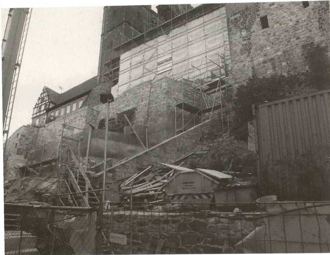
Quedlinburg, so-called Schlossberg, southern wall underneath the convent church during repairmeasures, October 2004 (photo: A. Hubel)
