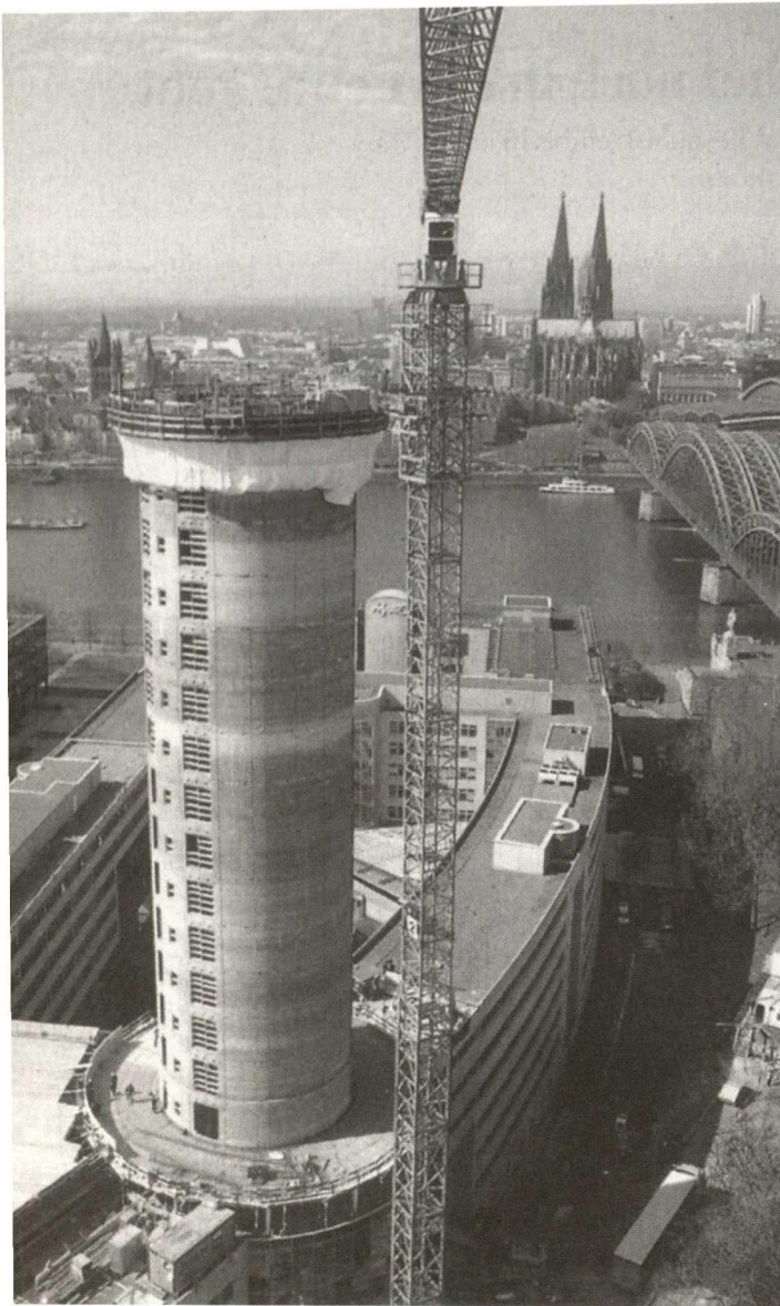
Cologne, the RZVK building during construction
