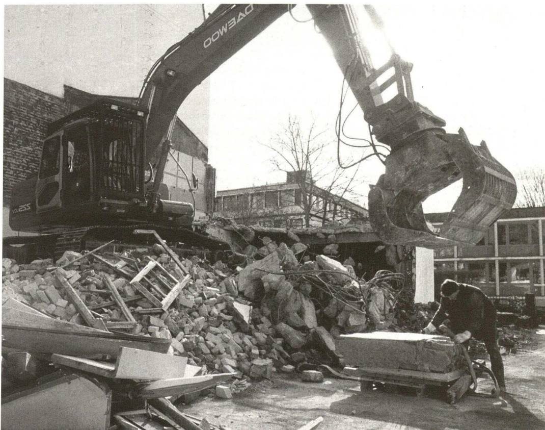
The demolition contractor rescues a remaining piece of wall with traces of the Gesamtkunstwerk
