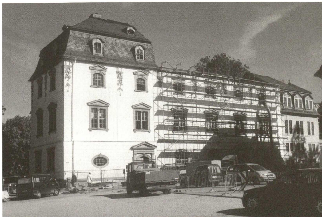
West facade with scaffolding for temporary roof (photo: J. Seifert)
