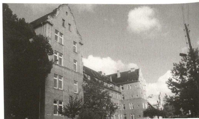
Quedlinburg, former infantry barracks, erected in 1909, buildings in Gneisenaustasse, October 2004 (photo: A. Hubel)
