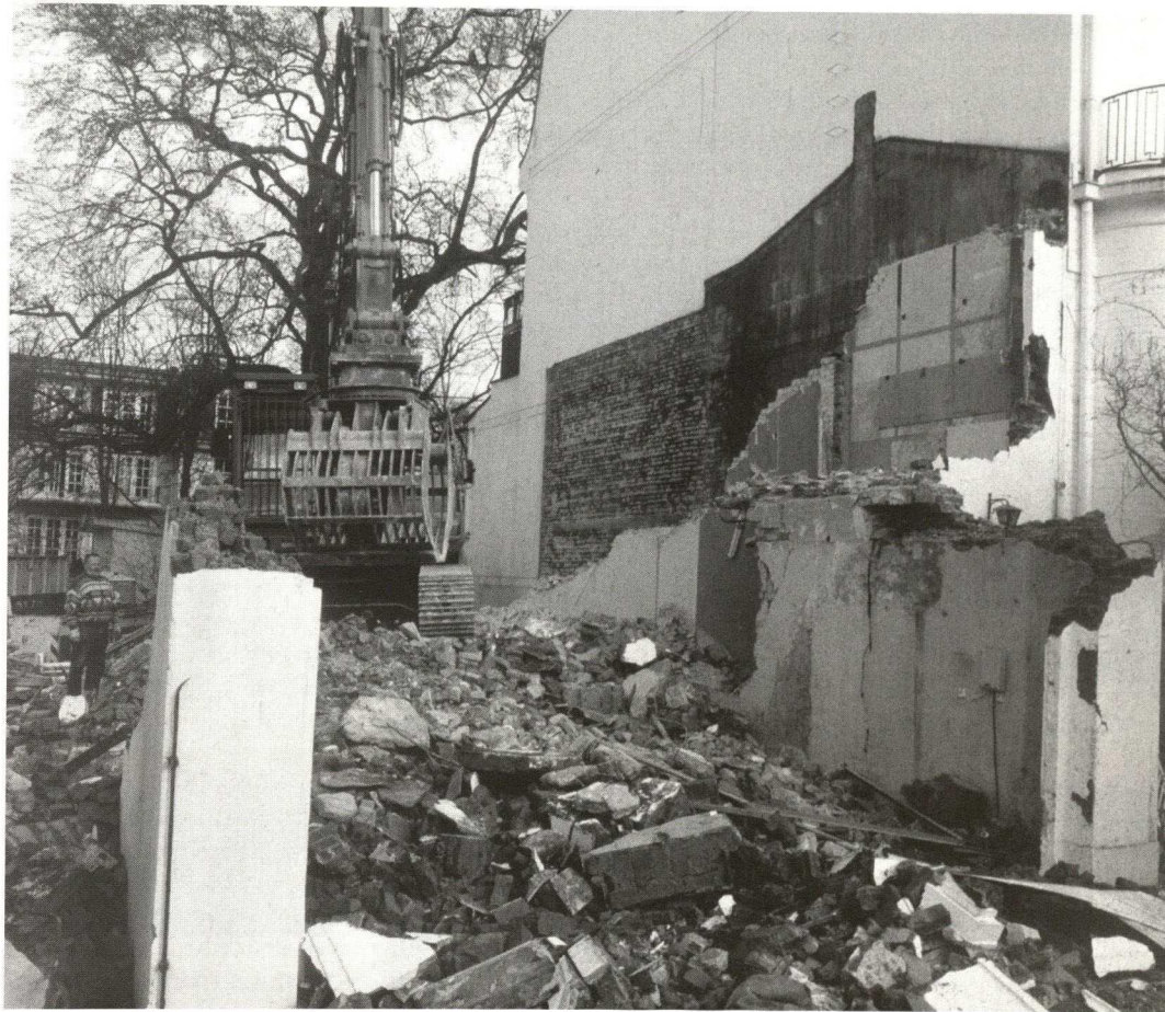
Demolition of the museum, on the remaining wall painted sections
