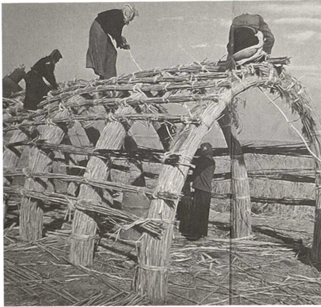
Reeds house under construction
