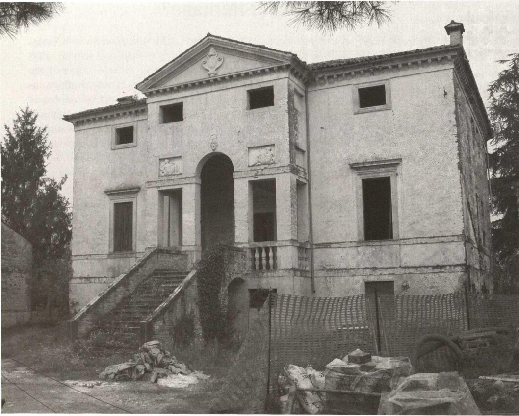
Villa Forni-Cerato in Montebelluna near Treviso, a building by Andrea Palladio (1541-2). A piece of World Heritage in an increasing state of decay (leaking roof, no windows, the dilapidated interior with endangered wall paintings).
