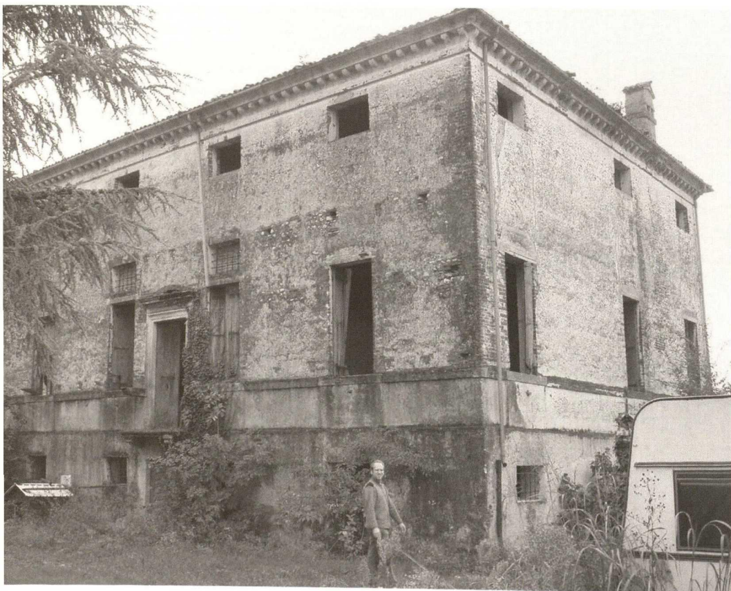
Rear of the Villa Forni-Cerato
