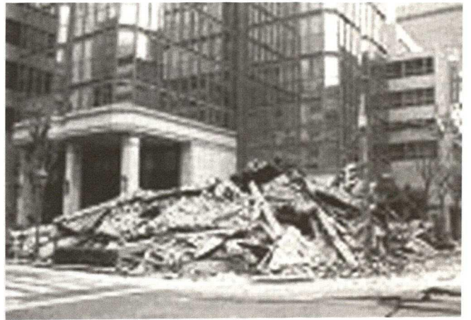
Kyokoryuti 15 banken, destroyed by earthquake
