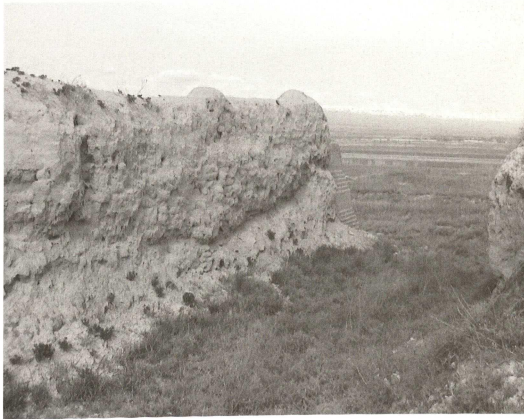
The mudbrick cella wall from south
