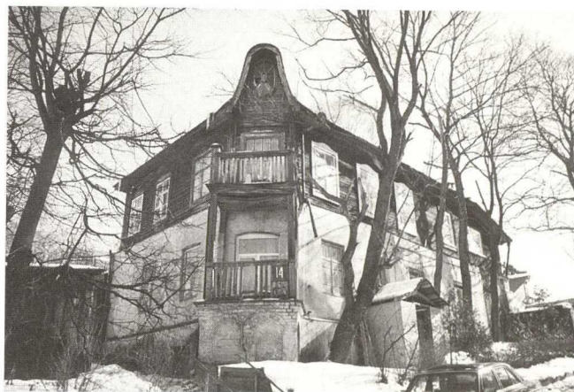
House in Pavasario Street
