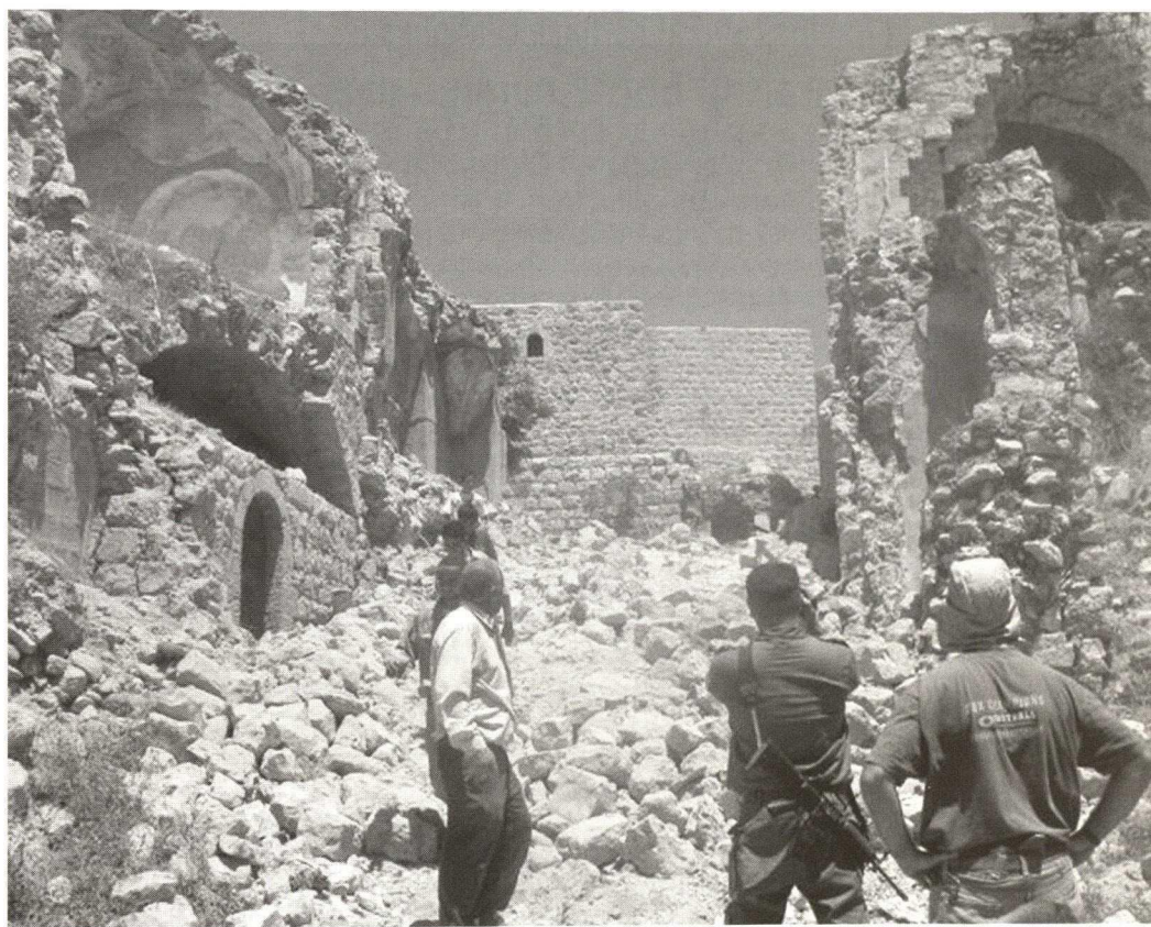
Destruction of Mamluk-era houses for settlers' road through Hebron's Old City
