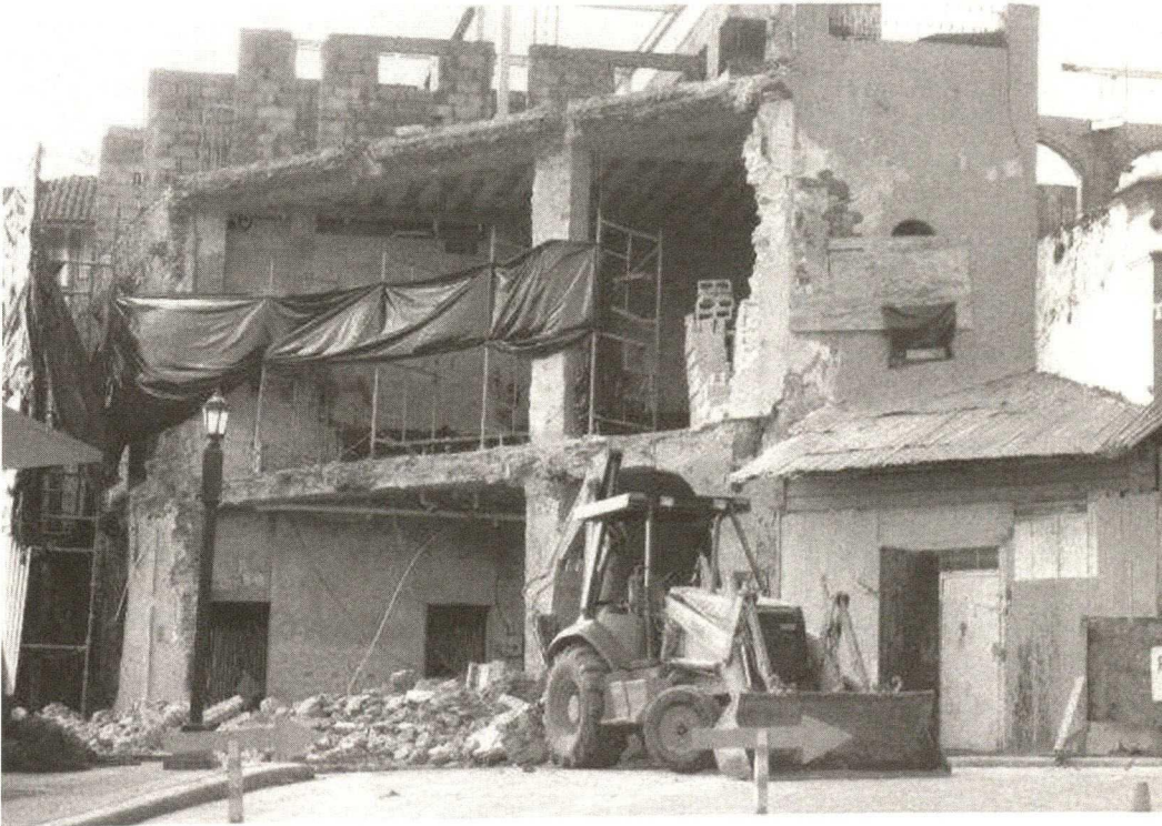
The demolished facades covered in plastic
