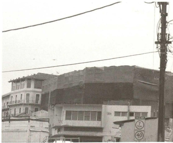
The demolished facades covered in plastic
