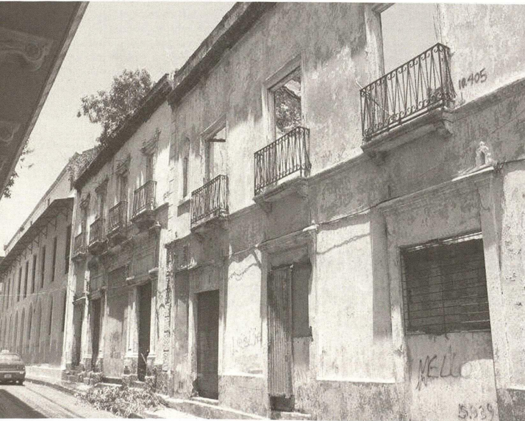
8th Street, facade (demolished)
