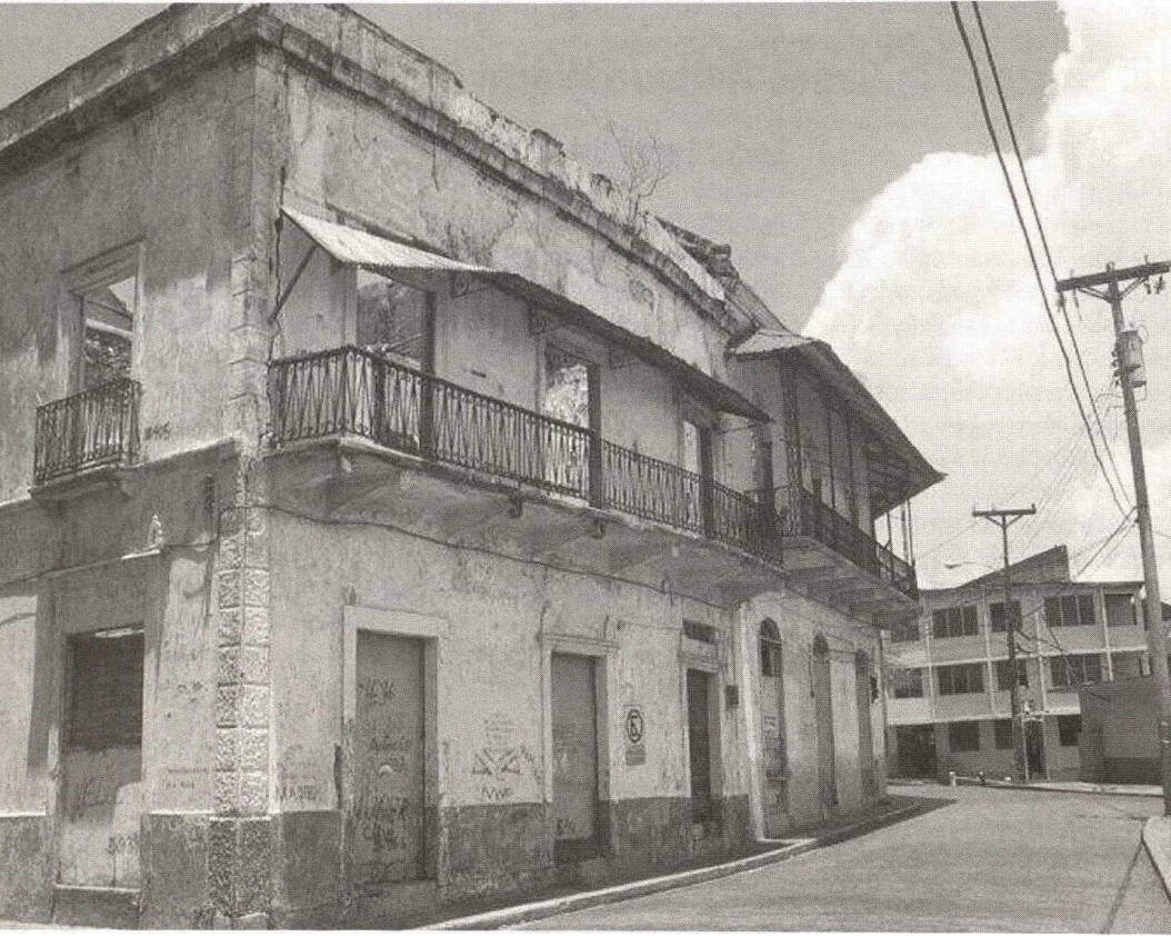
Ave. Eloy Alfaro, facade (demolished)
