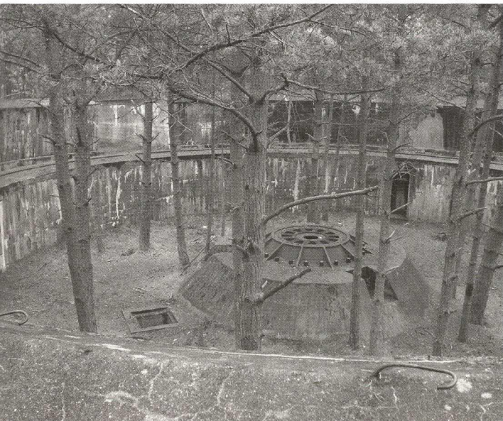
Schleswig Holstein Battery on Hel Peninsula, an example of a German military structure from World War II
