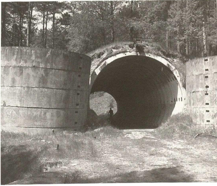
Brzeznica, near Borne Sulinowo, example of a Soviet military structure for missiles from the Cold War
