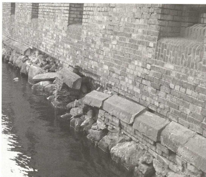
Vistulamouth Fortress in Gdansk, the brick bastions in need of conservation work
