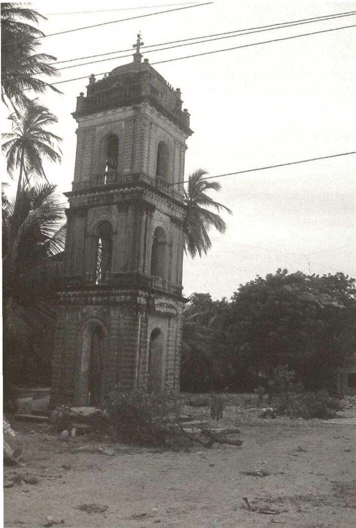
Church in pt. Pedro that has survived the tsunami
