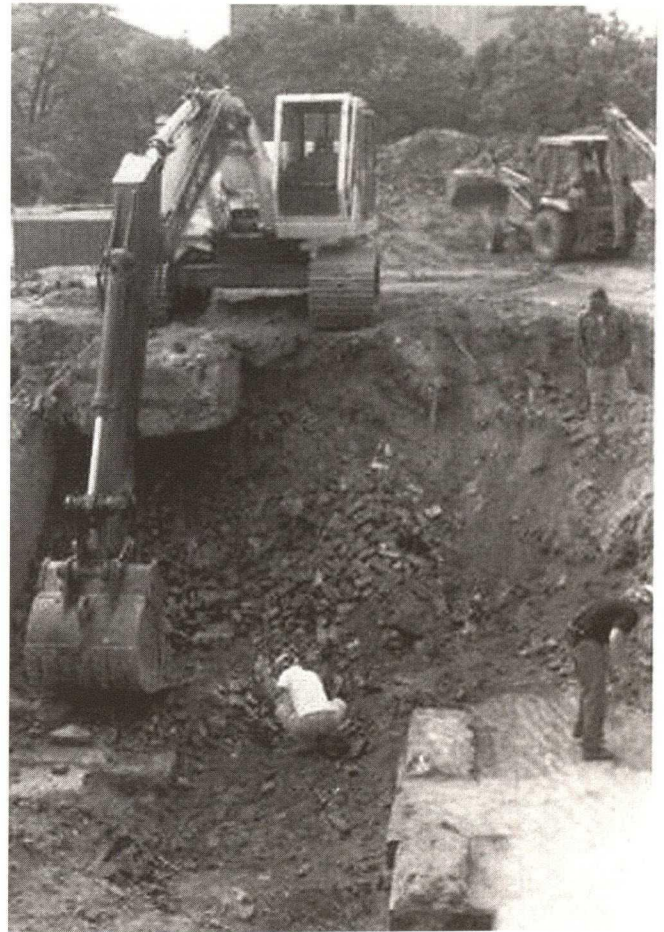
Excavation at Independence Park Visitors Centre, Philadelphia (photo: NPS, Jed Levin)
