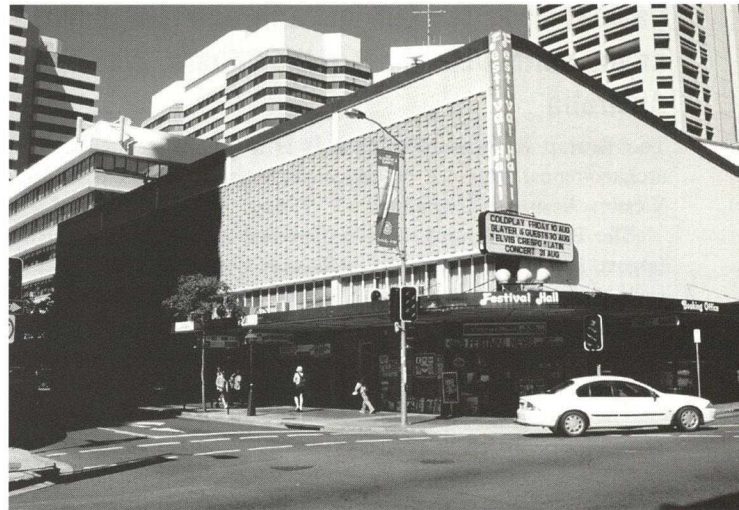
Festival Hall: Corner of Albert and Charlotte Streets, Brisbane, August 2001 (Qld Environmental Protection Agency file ref. 602154)
