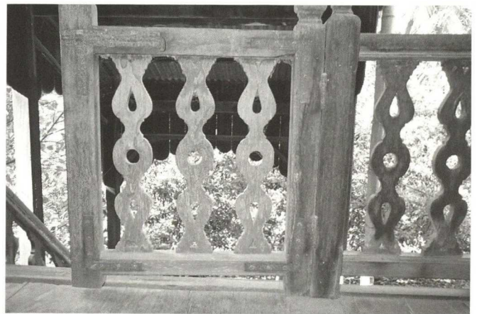
Guardrail, house in Battambang
