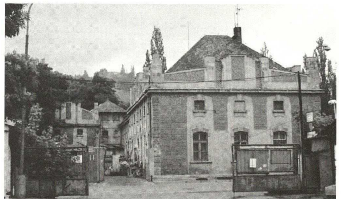
Ice-making plant, Prague – Bráník: present-day condition
