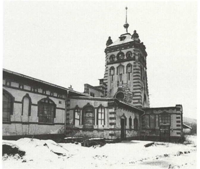
Ice-making plant, Prague – Bráník: present-day condition
