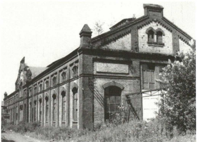
Workshop building of the coking plant Karolina, Ostrava, North Moravian Region
