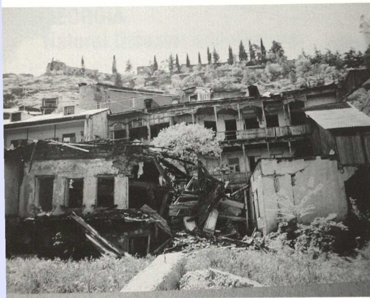
Residential buildings after the earthquake
