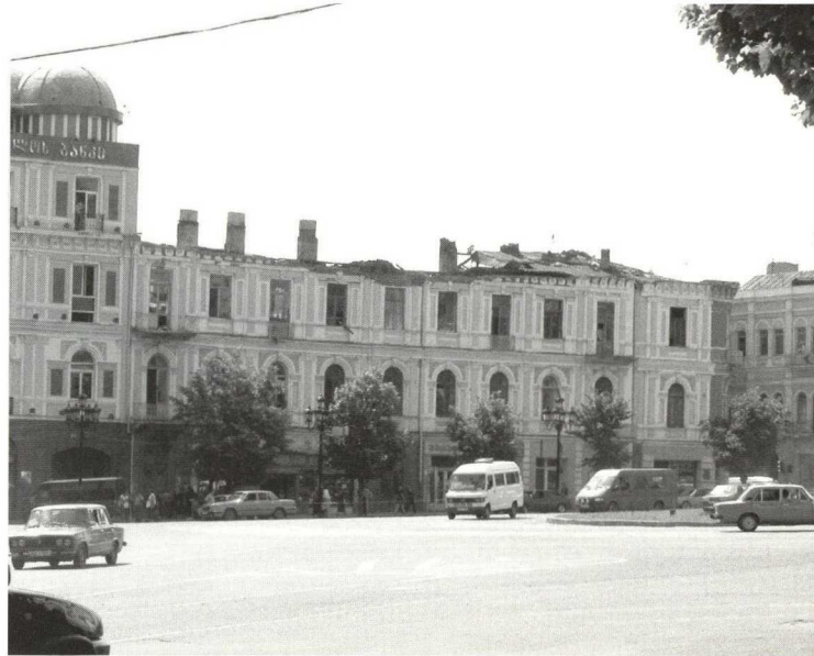
Damaged listed building on the Liberty Square destined for demolition by the city authorities
