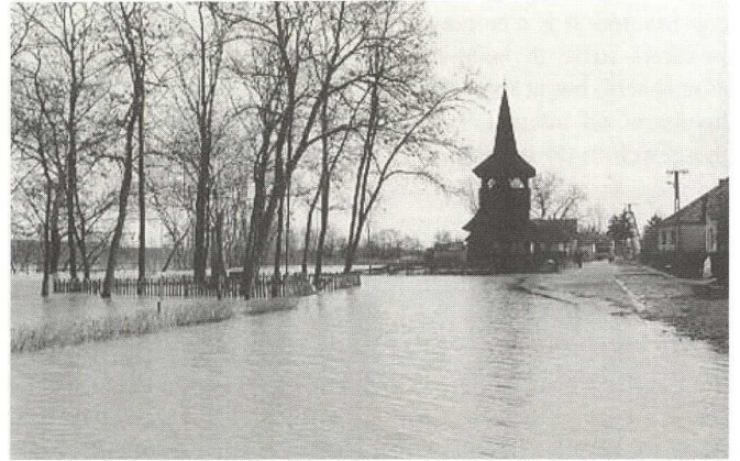
Tákos is flooded (Photo: István Szatmári)
