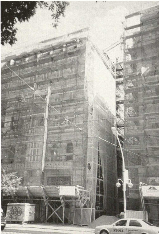
Façadism of another Budapest hotel under construction
