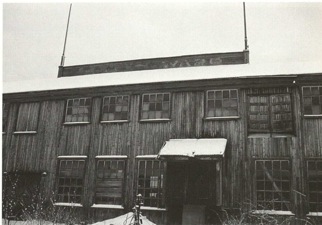
An early 20th-century timber merchant warehouse in Skien, County of Telemark, on the demolition list
