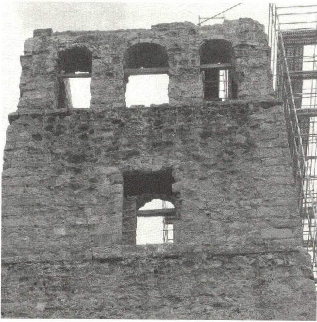
Cathedral Tower, Old Panama. National Heritage (erosion by winds and saltness, Nov. 2002).
