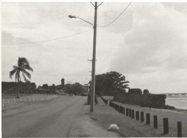
Ensemble of Old Panama. Vehicular road in the middle of the historic centre to be relocated (Nov 2002).
