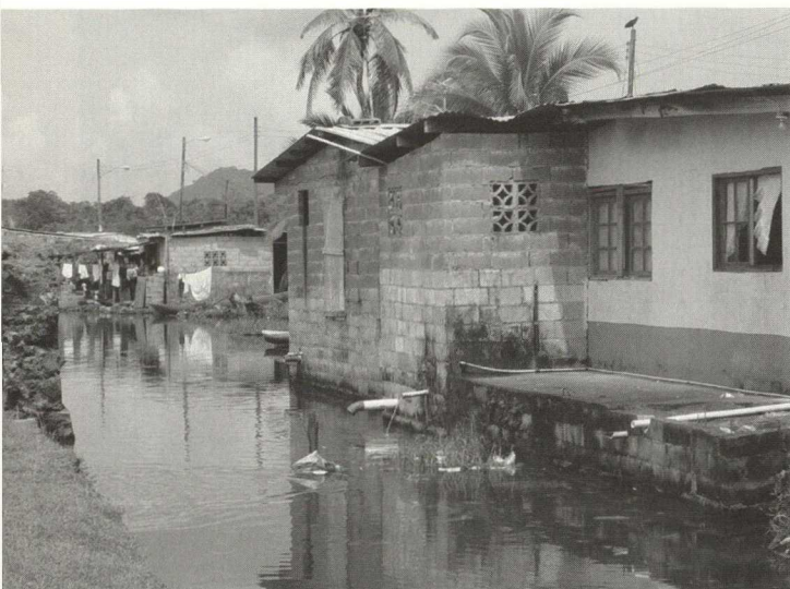
Fort of San Geronimo, Portobelo. Uncontrolled, improvised settlement adjacent to the heritage features (Nov 2002).
