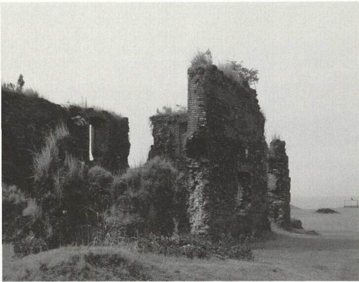
Castle of San Lorenzo. World Heritage (deterioration through lack of maintenance, Nov. 2002).
