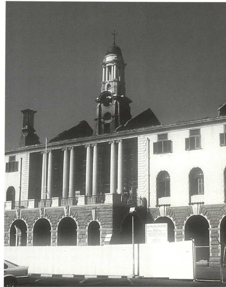
Pretoria's main railway station designed by Sir Herbert Baker and built in 1910–1912. This photograph was taken a few days after the destruction of the roof through fire on 19 February 2001. The fire was started by an angry mob of railway commuters who vented their frustration because of trains running late at evening rush hour. The building has since then been restored. (Photo: R.C. de Jong)
