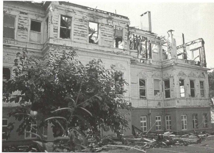
Late 19th-century timber palace on the Bosphorus, Istanbul, devastated by fire. Electrical installations in historic buildings are often the cause of such losses. Used as a public school, the building was suffering from lack of funds for its maintenance.
