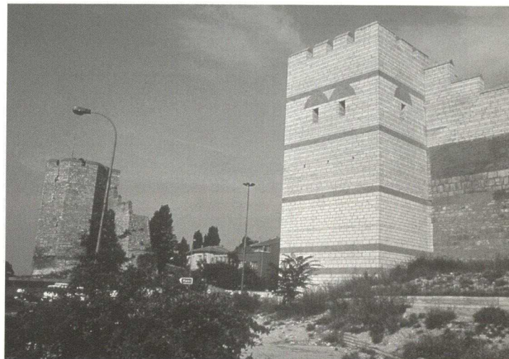
Tower 89 of the Theodosian Wall had suffered from the earthquake in 1999 (see Heritage at Risk 2000 for a photo of the damaged state). The vestiges were not enough for a proper reconstruction. A new tower has been recreated, reducing the significance and legibility of the ancient remains.
