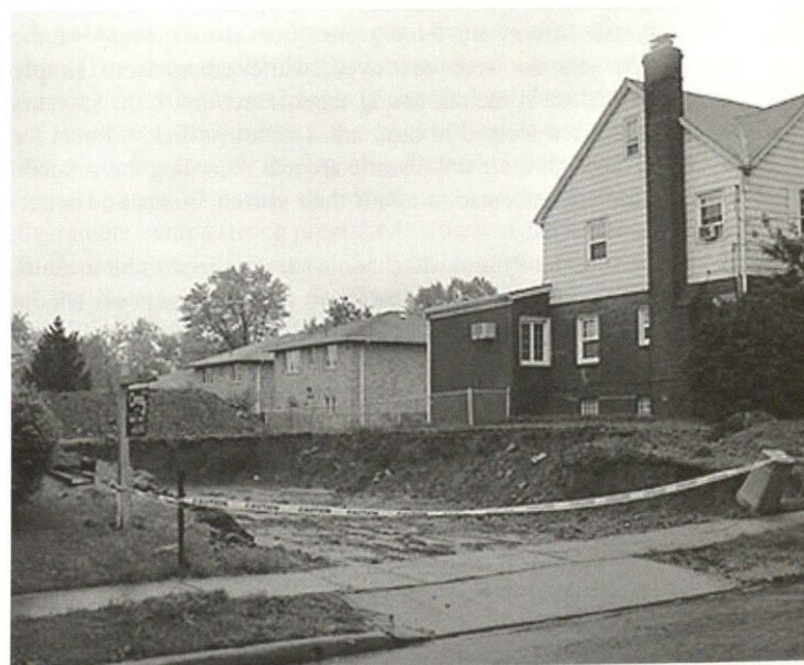
Teardowns in Historic Neighborhoods, Bergen County, New Jersey (Photo: Adrian Scott Fine, National Trust)
