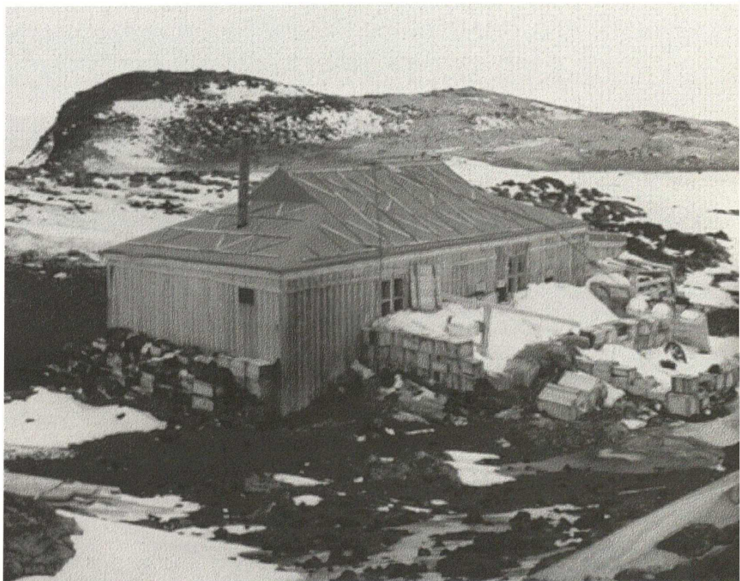
Insulation for this prefabricated building was improved by stacking boxes of supplies around the outside walls and filling the space between with volcanic scoria. Cape Royds, Antarctica. (Photo: P. Chaplin)
