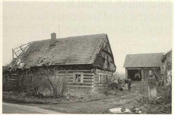
Studeňany, land-register No. 45, District of Jičín - a dilapidated timbered farm before its complete demolition
