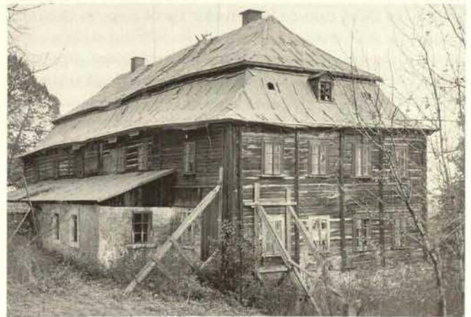
Krásná, land-register No. 10, District of Jablonec nad Nisou - a massive timbered house built in the mid-18th century, its present state being critical
