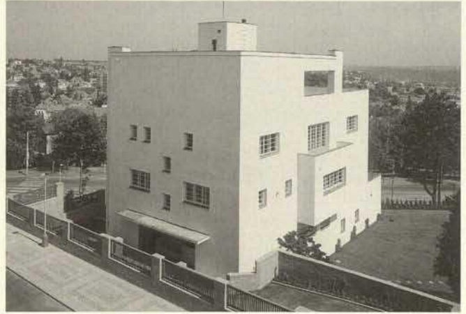
Prague 6 - Střešovice, Müller's Villa, state of the exterior after renovation
