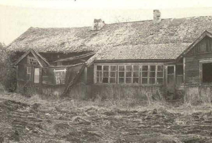
Old farmhouse in decay
