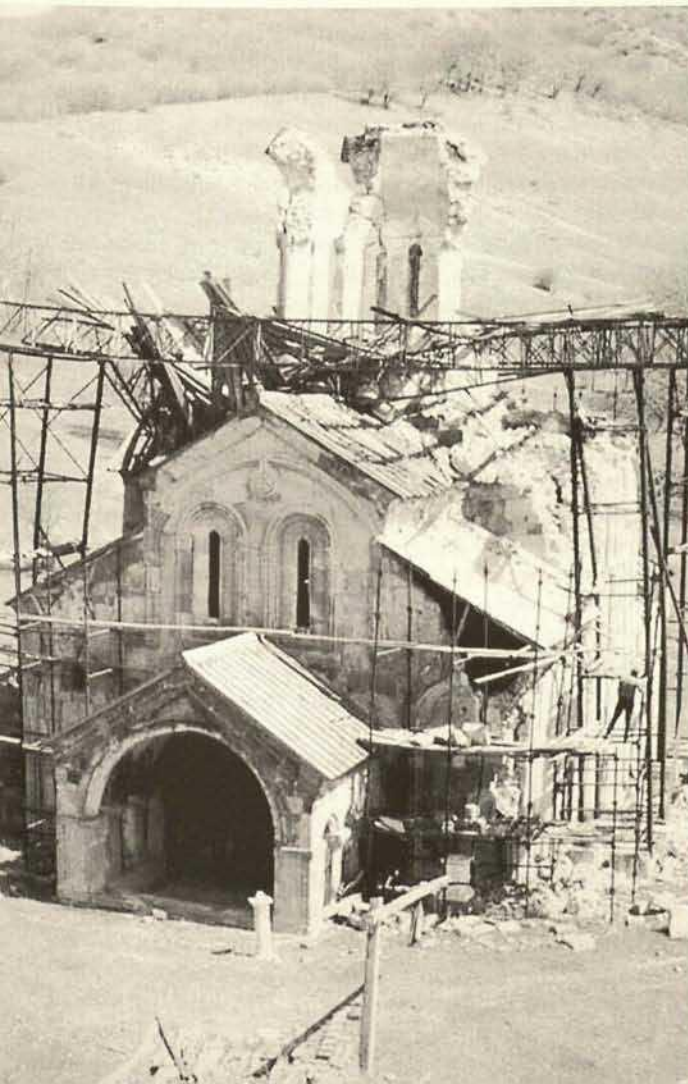
Ikorta church of the Archangel after the earthquake
