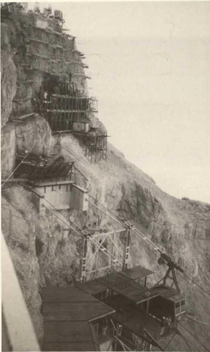
Masada, construction of a new cable car
