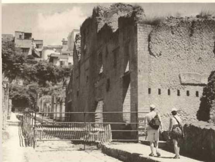
Herculaneum, 5th Cardo with street front of the vestibule of the Palestra in danger of collapse
