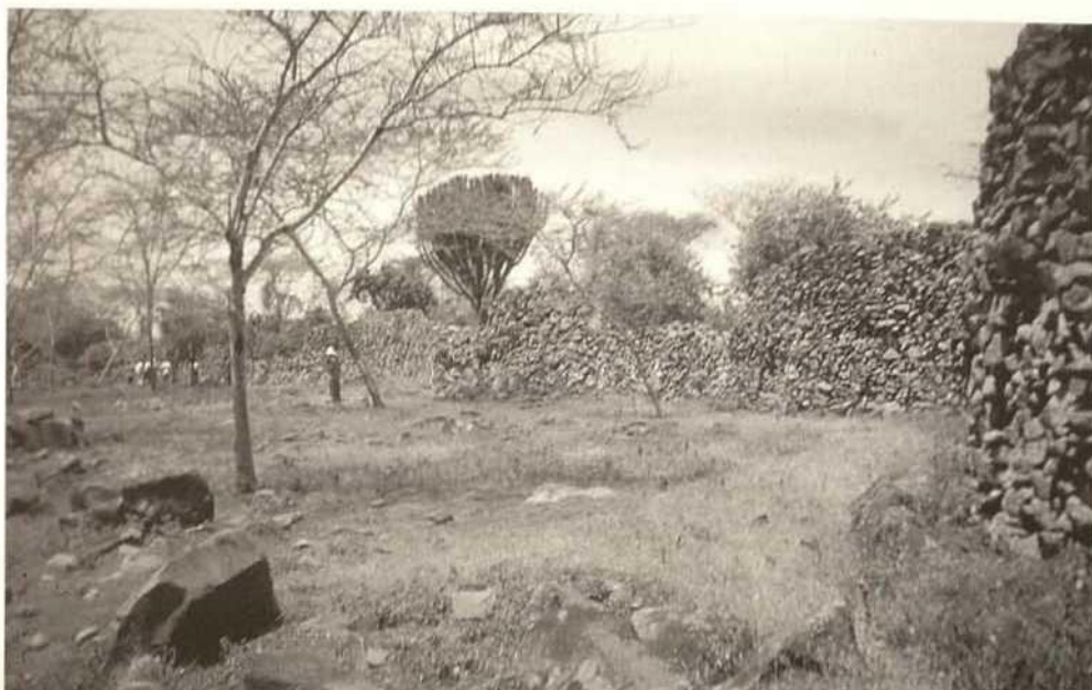
Thimlich Ohinga, view during the wet season. Note the collapsed wall in the background.
