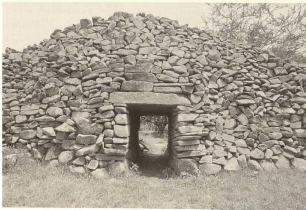
Entrance of dry-walling enclosures of Thimlich Ohinga in South Nyanza. Note the similarities with Great Zimbabwe.
