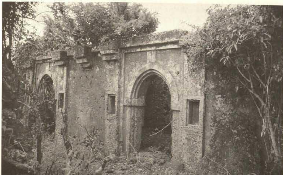
Mwana, remains of a residential house
