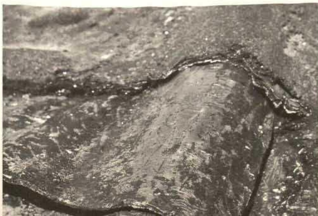
Lead plates covered with bituminous felt
