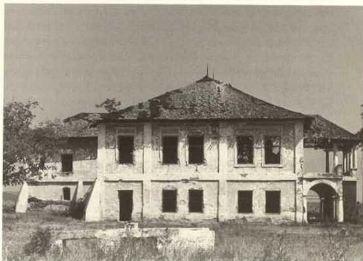
Strejesti, district of Olt, the Buzescu-Darvari mansion, side façade, state of 1999
