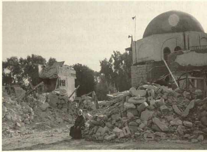
Zuqaq al-Zukhra, extra-muros, destruction of an old quarter for a new hotel
