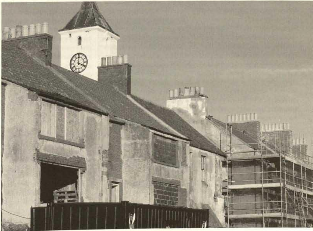
West Wemyss village, Scotland, during restoration
